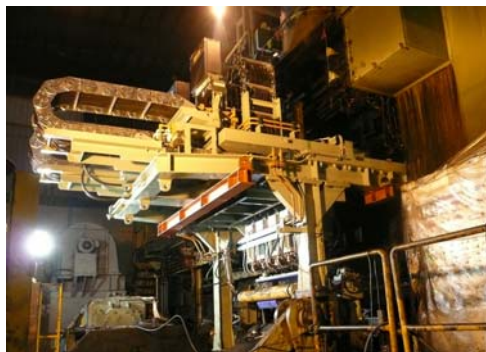
Figure 11. Zoom device in erection
