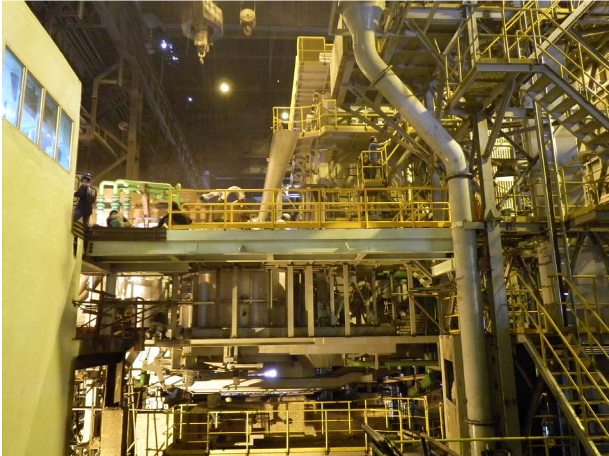
Fig-11: State under construction (view from tapping side)
